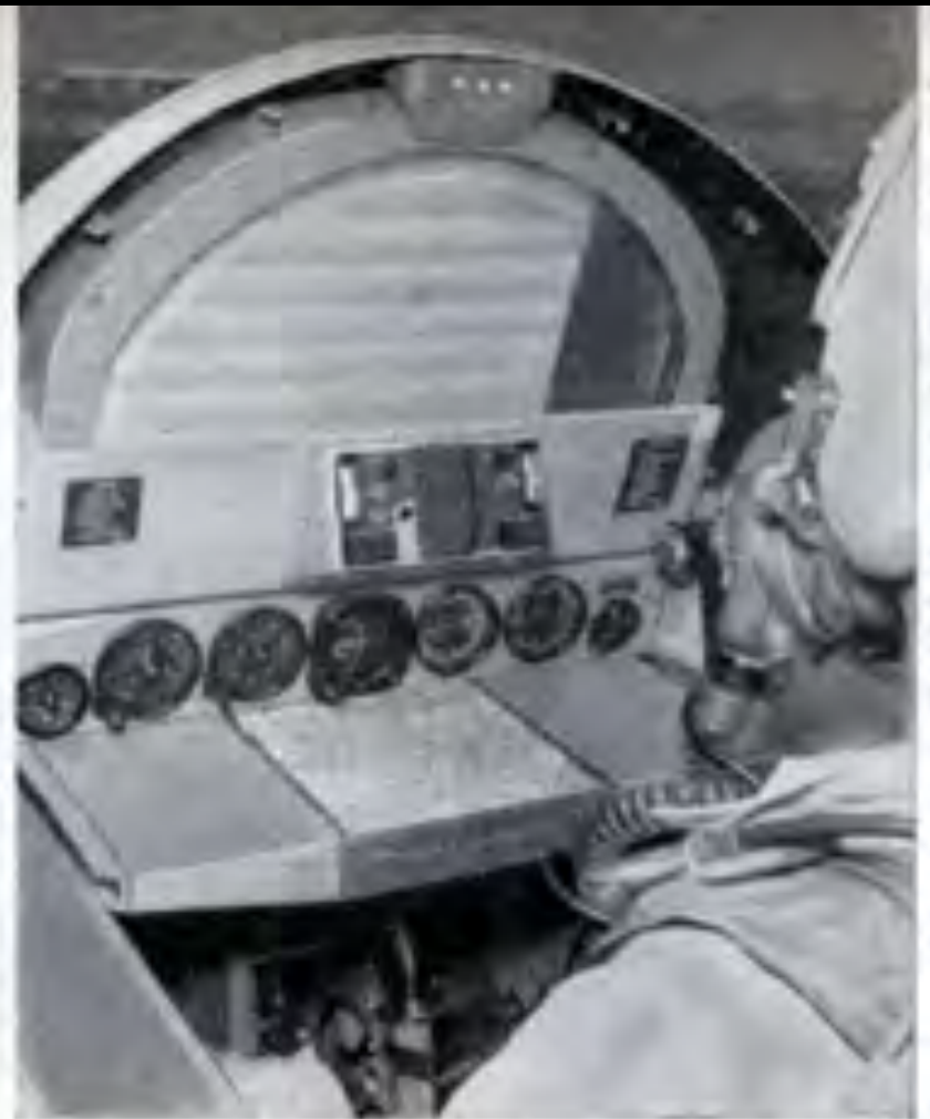
Used in airplane cockpit, picture of area in which pilot is flying appears on TV tube in front of him
