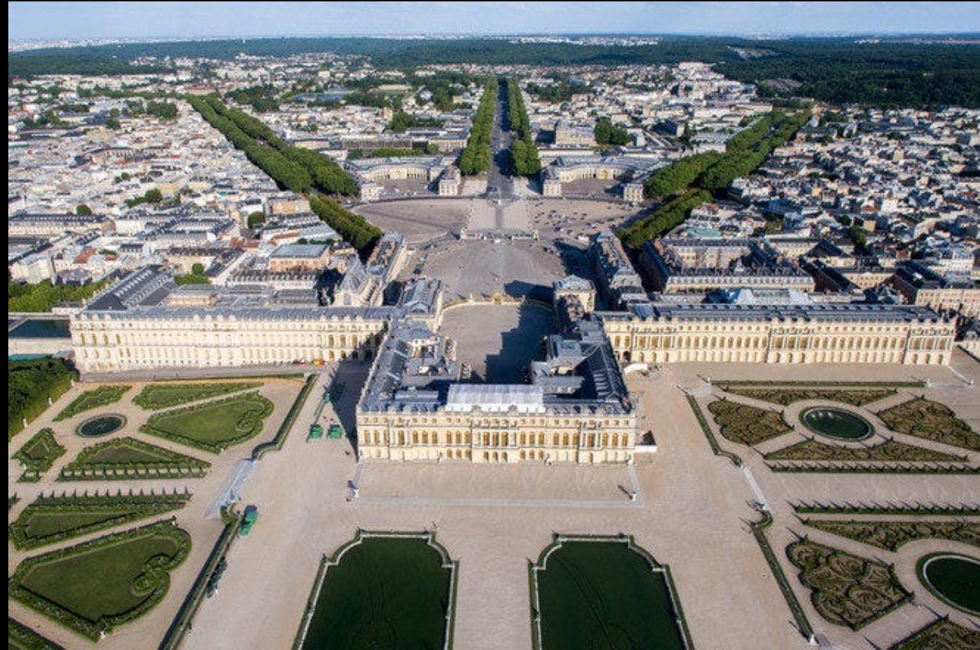
Palace of Versailles, Architects: Philibert Le Roy, Louis Le Vau, Jules Hardouin-Mansart, 1670-1700
