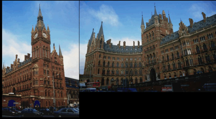
William Henry Barlow and George Gilbert Scott, St. Pancras Station (and Midland Hotel), London, details of southeast corner and south (main entrance), 1868-1874
