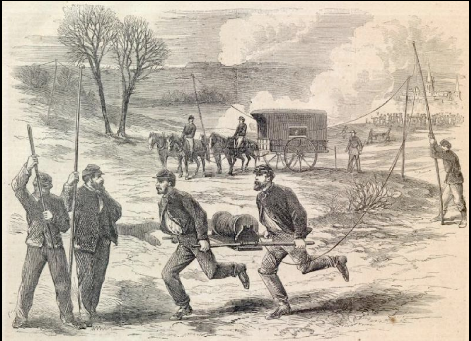
Erection of first telegraph lines 1840s
