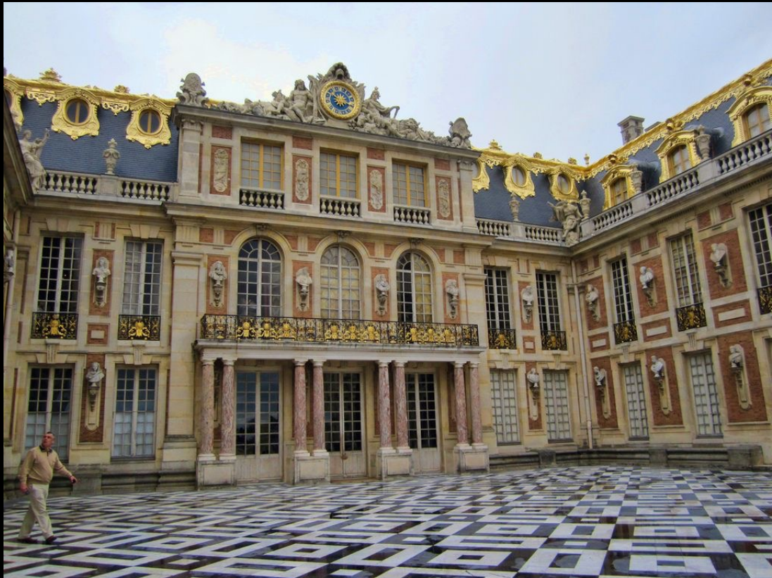
Detail of Palace of Versailles, Roof designed by Jules Hardouin-Mansart
