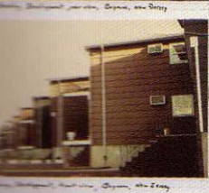
Two-story house is usually called "colonial". It consists of contiguous boxes with one slightly higher elevation at a "split level". Such a differentiation is advantageous to the basic structure (with the possible exception of the split level whose plan supplies construction on discontinuous ground levels).
