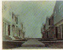
Center Court, Bahama, Development, Jersey City, N.J.
